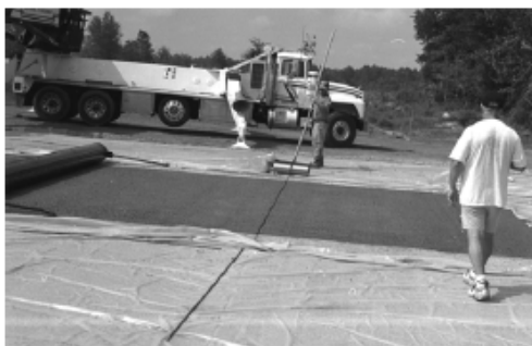
Fig. 8.14—Example of use of reinforcing bars to hold down curing material.
