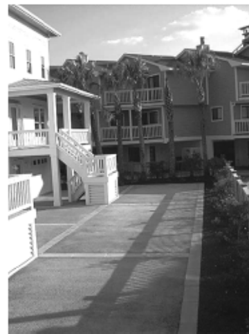
Fig. 3.1—Parking lot built with pervious concrete pavement.
