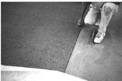
Fig. 8.10—Edging pervious concrete to improve appearance of corners.
