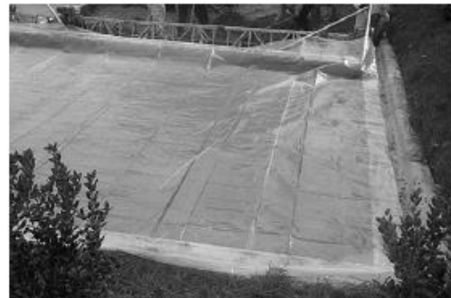
Fig. 8.13—Demonstration of curing with plastic sheeting immediately after compaction
