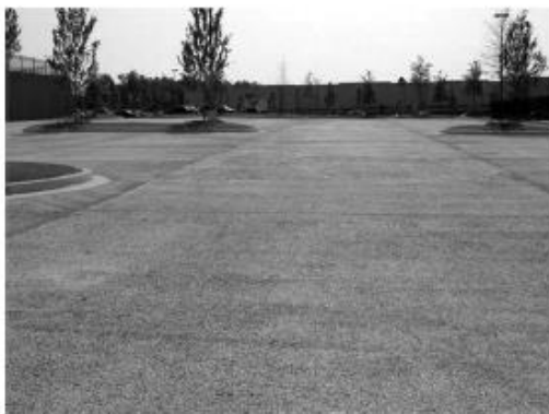
Fig. 12.3—Pervious concrete parking lot.
