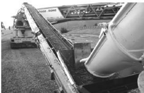
Fig. 8.2—Use of conveyor to place pervious concrete.
