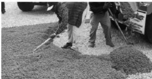
Fig. 8.3—Raking pervious concrete to rough elevation.
