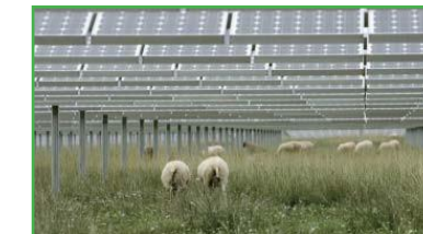
Farm solar generation system
