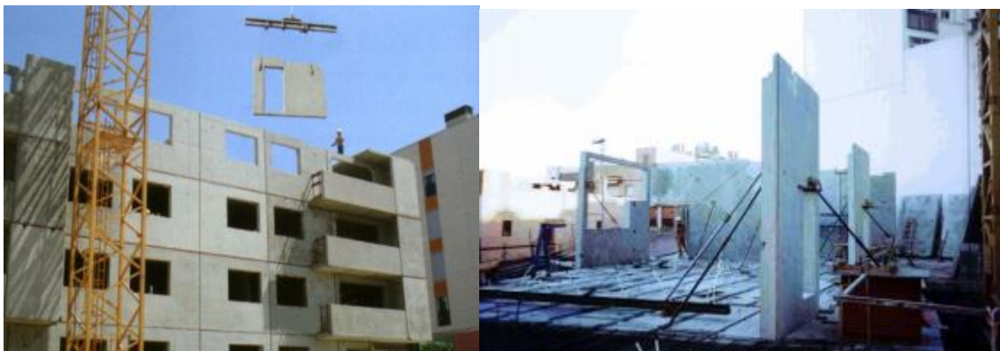
Fig. 10 BSCP (Building System with Concrete Panel)
